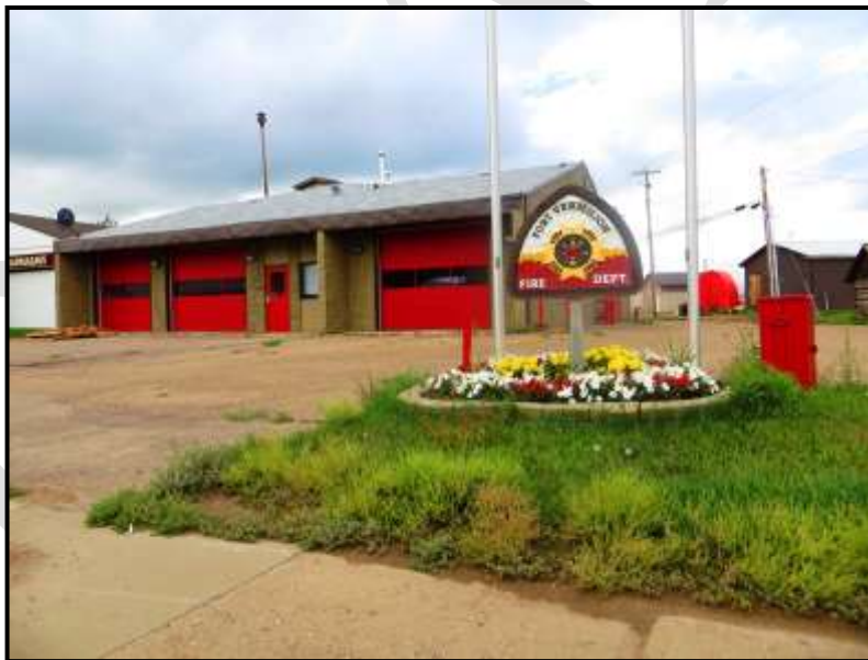
Fort Vermilion Fire Station
